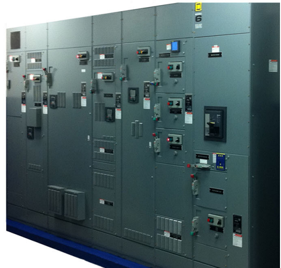
Example Fully Integrated Motor Control Center
